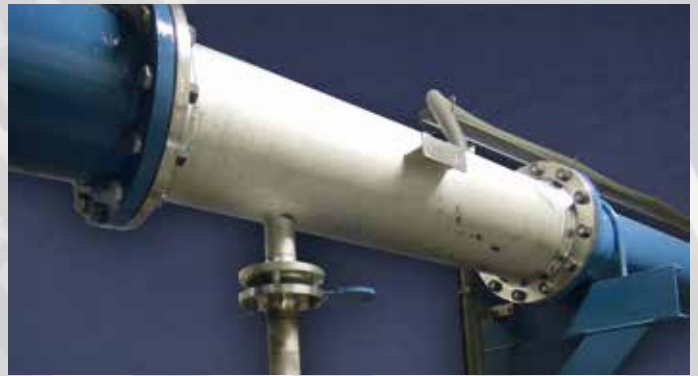
Ammonia mixer for power plant
